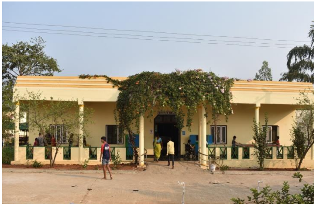
Kitchen after renovation
